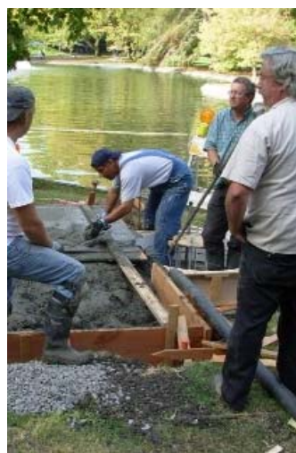
Pouring concrete for the Holocaust and Genocide Memorial Grove Project at the Lakes on the Sonoma State campus (10/08)
